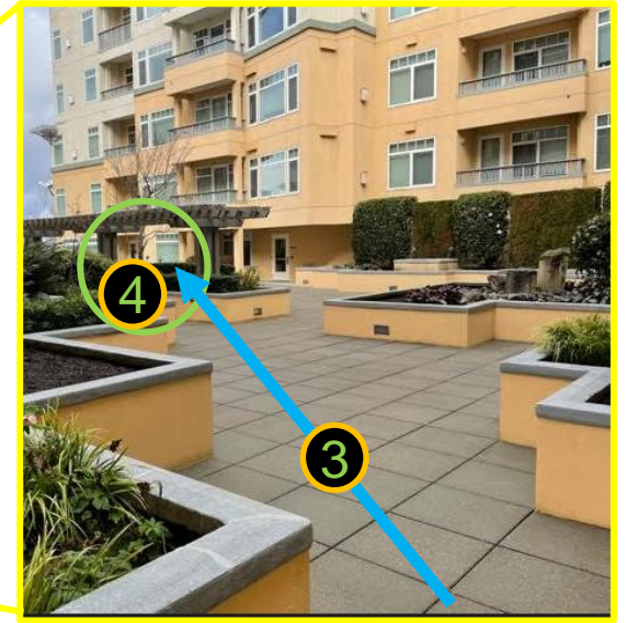
Clubhouse (Back Left Wall)
